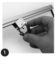
Carefully open clips and press into position along profile length (min 3 clips per metre or every 500mm/20").
